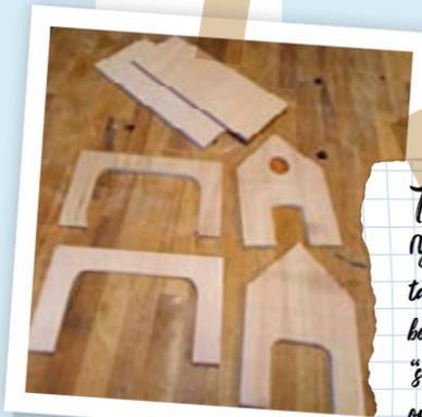
**2** Cut the basic parts to size. Make sure that the dimensions of the opposing walls are identical. Cut out further openings as needed.
